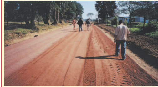
Immediately after the Otta Seal aggregate has been applied. The seal looks like a gravel road at this stage. But with time, the single Otta Seal will "bed down" and a bit premix type appearance will appear. (South Africa).
