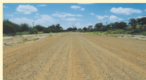
Otta Seal surfacing, 2 - 3 days after construction, and where traffic has been allowed using the surfacing immediately after construction. (Botswana).
