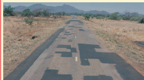
On pavements that have deteriorated badly, an Otta Seal, because of its durability (high bitumen content and low viscosity binders which make the Otta Seal very flexible) is well suited as a reseal. (Malawi).
