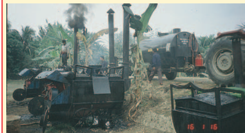
At the Environmental trial Road at Faridpur, the bitumen was both cutback and fluxed in order to give the correct binder consistence. This was successfully carried out by simple but appropriate methods. (Bangladesh).
