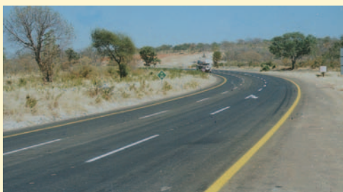
After some months the Otta Seal with a sand cover seal are fully settled and shows excellent appearance. (Botswana).
