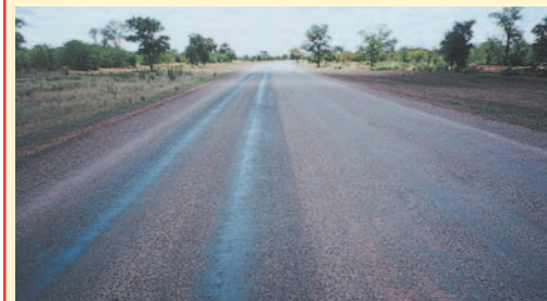
Some bleeding in localised areas and in the wheel paths form a normal part of the curing process. Severe bleeding can be rectified by sand or additional aggregate rolled into the bleeding areas. (Botswana).
