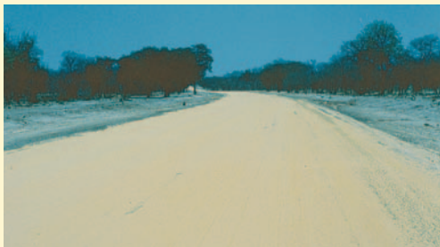
Over application of sand is essential when applying a sand cover seal on top of a single Otta Seal. (Botswana).
