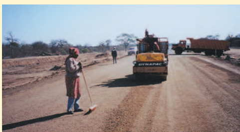
One pass with a static tandem steel roller will improve the embedment of the larger aggregate.
