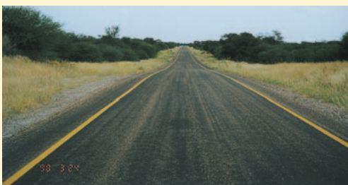
After some months in service the Otta Seal “beds down” and provide an uniform appearance. (Botswana).
