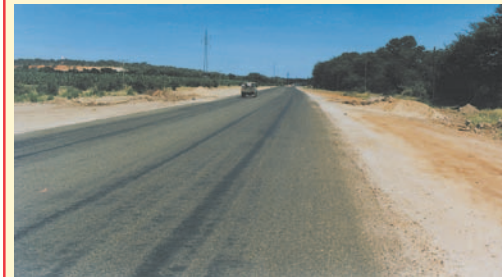
After a period of 8 - 10 weeks (traffic dependent), the Otta Seal beds down to produce the appearance of an asphaltic concrete premix. (Botswana).
