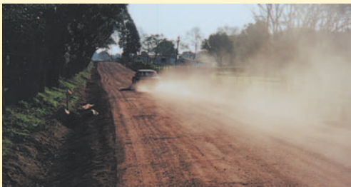
A newly laid Otta Seal (with a high fines content) will for the first 2 - 4 weeks give dust pollution. (South Africa).
