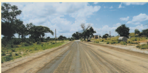
Correct aggregate application rate. (Botswana).
