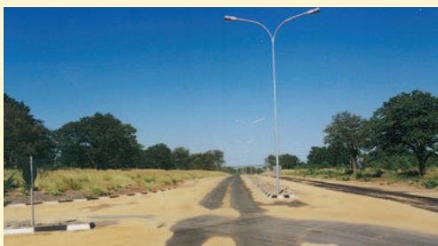
The sand blown off by traffic should be broomed back into the exposed areas until full embedment is achieved. (Botswana).
