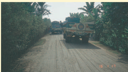
In the absence of pneumatic tired rollers, rolling of the Otta Seal can be done by loaded trucks following a pre-determined pattern of rolling. (Bangladesh).
