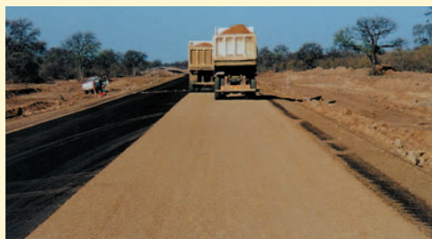
In the absence or in addition to pneumatic rollers, compaction can be successfully carried out by the use of loaded trucks following a pre-determined rolling pattern covering the entire surfaced area. (Botswana).
