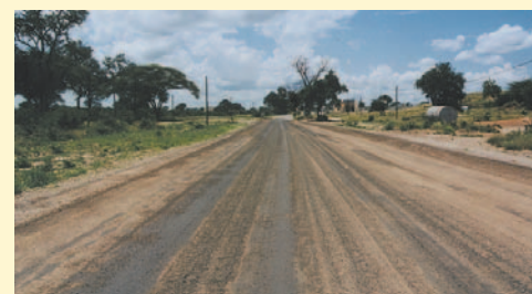
Aggregate that has been dislodged by traffic should be broomed back into the wheel paths. This to ensure maximum embedment of the aggregate into the soft binder. (Botswana).
