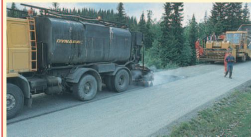
Otta Seals have been and is still extensively used in Norway. (Norway).
