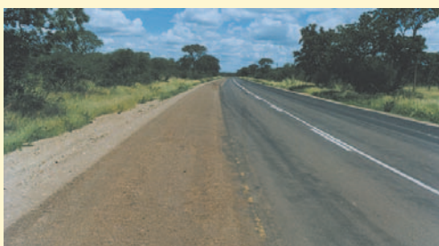
An Otta Seal will apparently show a significant difference visually between the shoulders and the carriageway. The traffic in the carriageway area works the binder upwards to the surfacing and hence, making difference in colour. This difference in colour will improve the traffic safety aspect. (Botswana).
