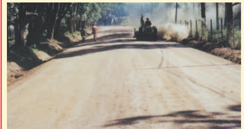
Preparatory work prior to sealing operation, clearing loose material from the base. (South Africa).
