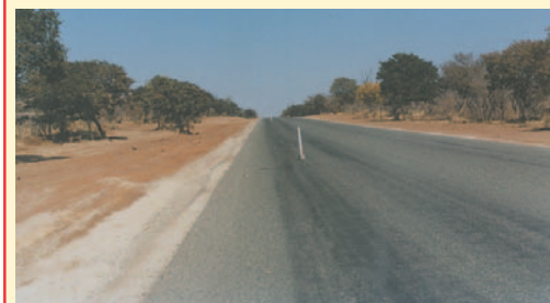
The Otta Seal should preferably be equally exposed to traffic over the entire sealed area as this will enhance an uniform appearance. This can be achieved by the use of traffic cones to direct the traffic in to areas that need trafficking. (Botswana).
